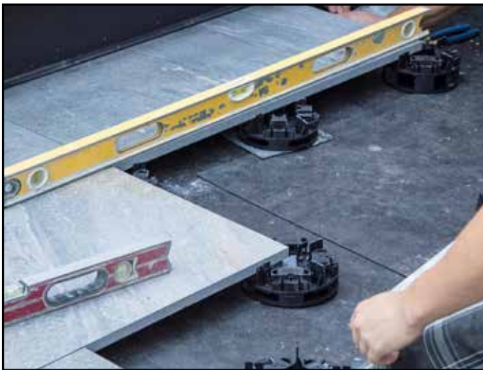
BlackJack OneStep Extenders provide height extension up to 4.13" (105mm).
