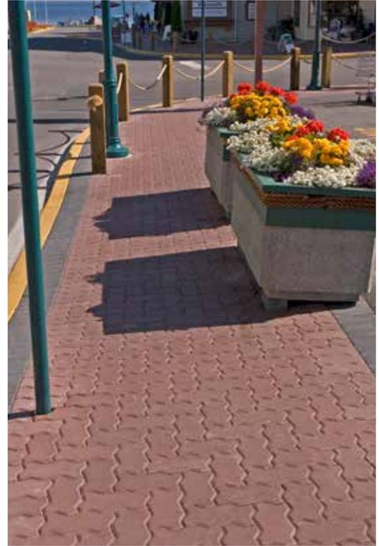
Our pavers are made with our unique **Face Mix** two layer process. In this process, the wearing surface of the paver is composed of uniformly graded hard, sharp granite aggregate, high cement content and a correspondingly high pigment content.
