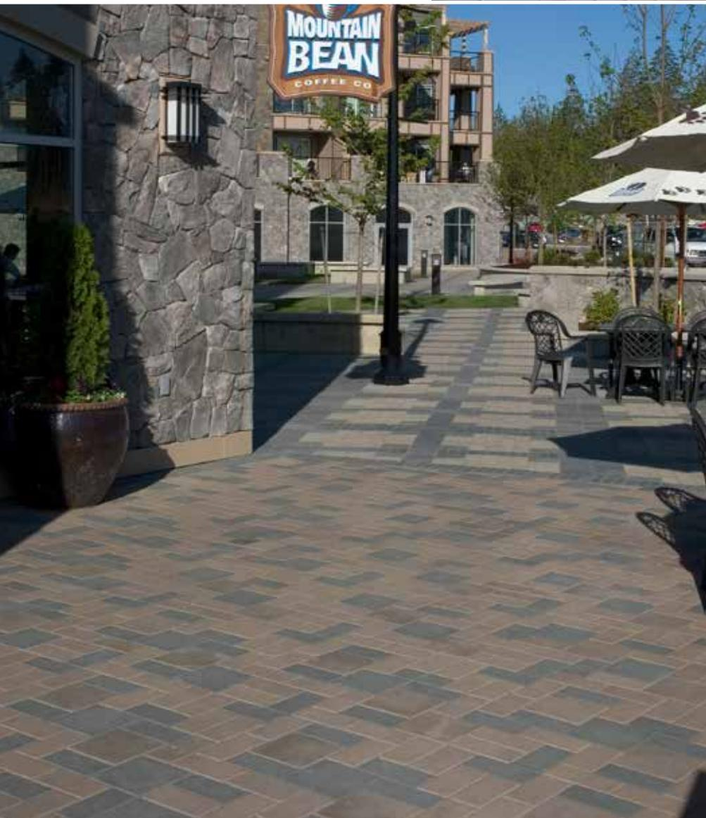
*Our pavers are made with the unique **Face Mix** two layer process. In this process, the wearing surface of the paver is composed of uniformly graded hard, sharp granite aggregate, high cement content and a correspondingly high pigment content. This results in a dense high strength surface, more intense color stability and greater abrasion resistance than traditional paving stones. The balance of the paver is composed of high strength compressed concrete.*
