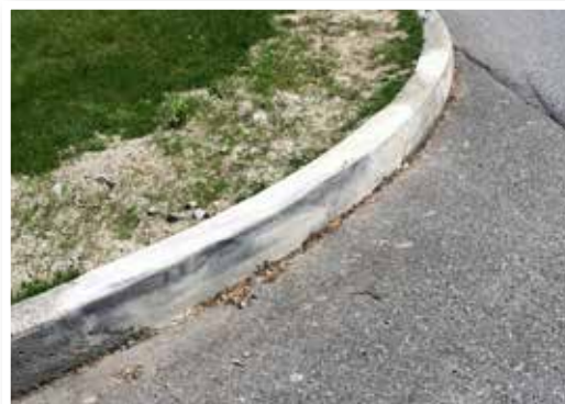
Unprecedented performance after months of continuous traffic abuse.
