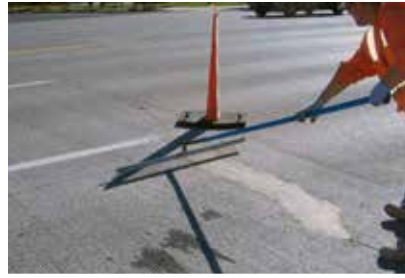
Cut a hard edge around damaged area
