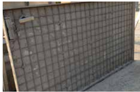
Old material is removed from panels
