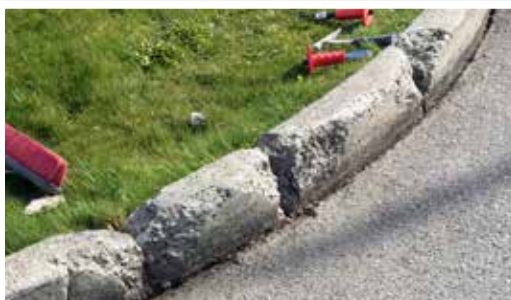
Damaged curb was repaired without deconstruction or forming.
