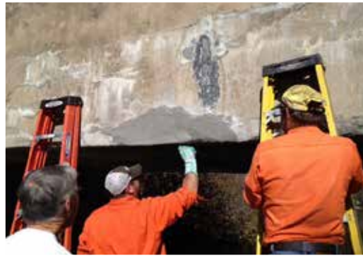
Repair should last a lifetime.
